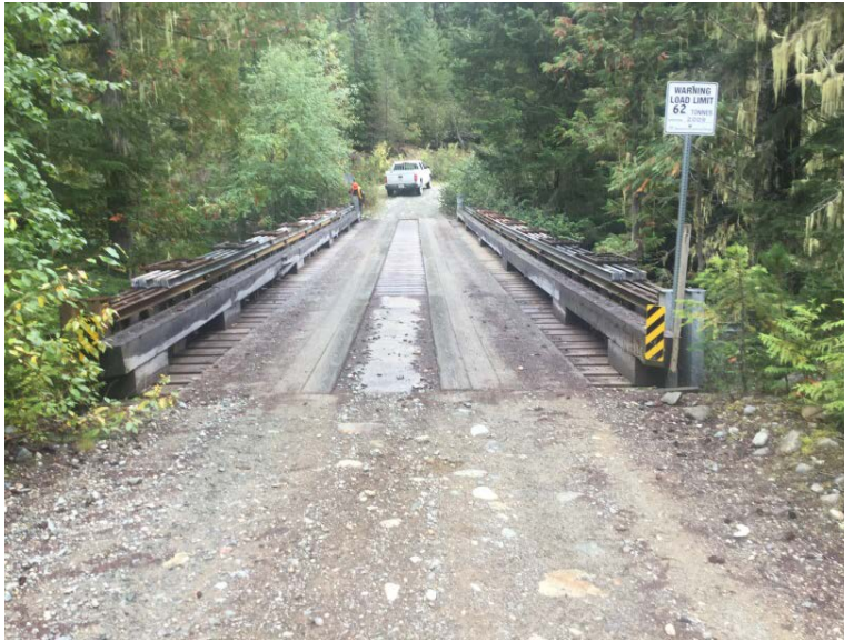
Approach from Right Bank when facing downstream
