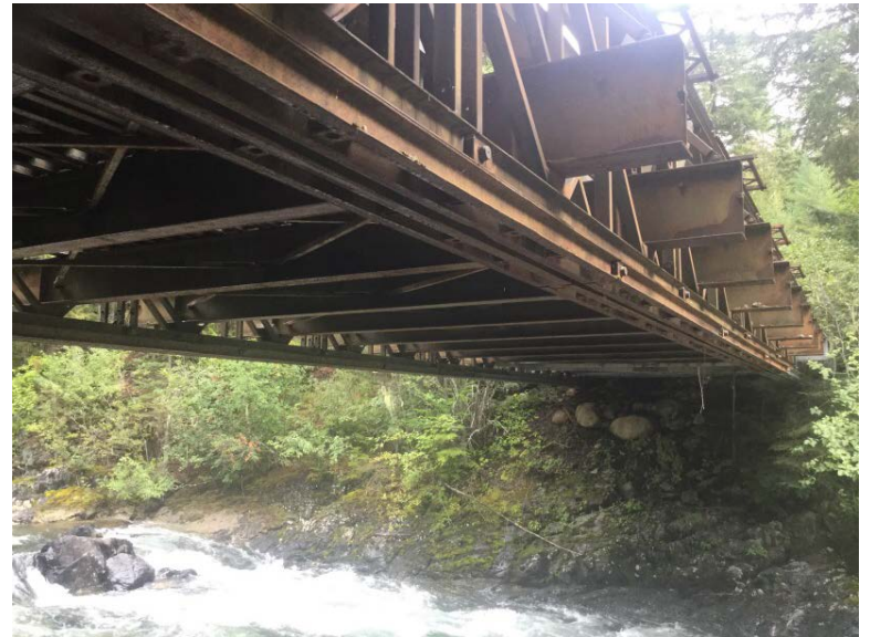
Left Bank Abutment when facing downstream
